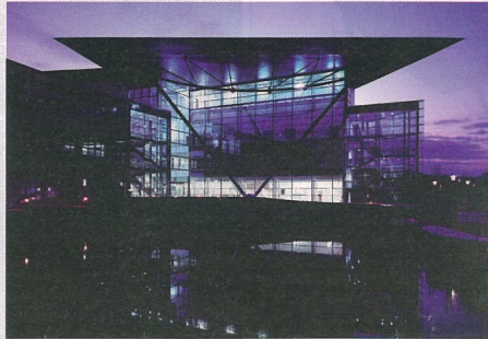
Construction of Broadway Malyan's Met Office in Exeter was aided by using Buzzsaw.
